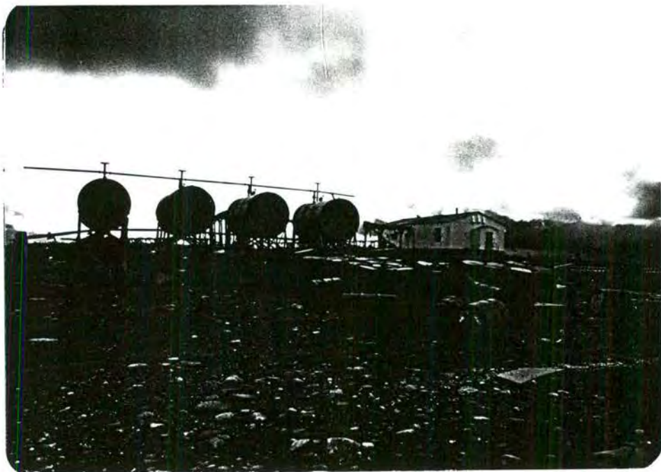
Photo 37: POL storage tanks and drums at Site 218.
