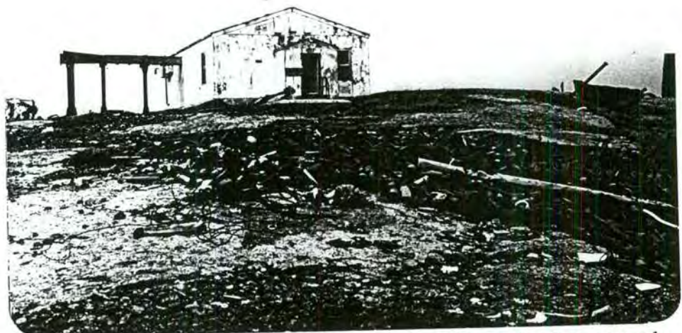
Photo 3: Doppler Detection Building, note litter in foreground.
