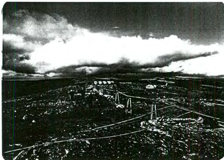
Photo 33: Pipeline to POL storage tanks at Site 221.
