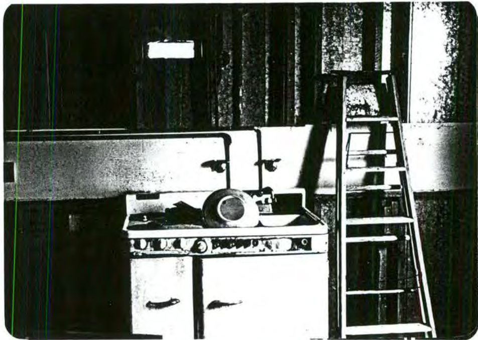
Photo 41: Interior view of kitchen at Site 215 with cabinets removed.
