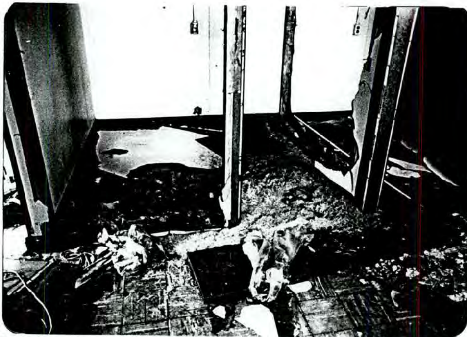
Photo 25: Extensive vandalism found in the Doppler Detection Building at Site 227.
