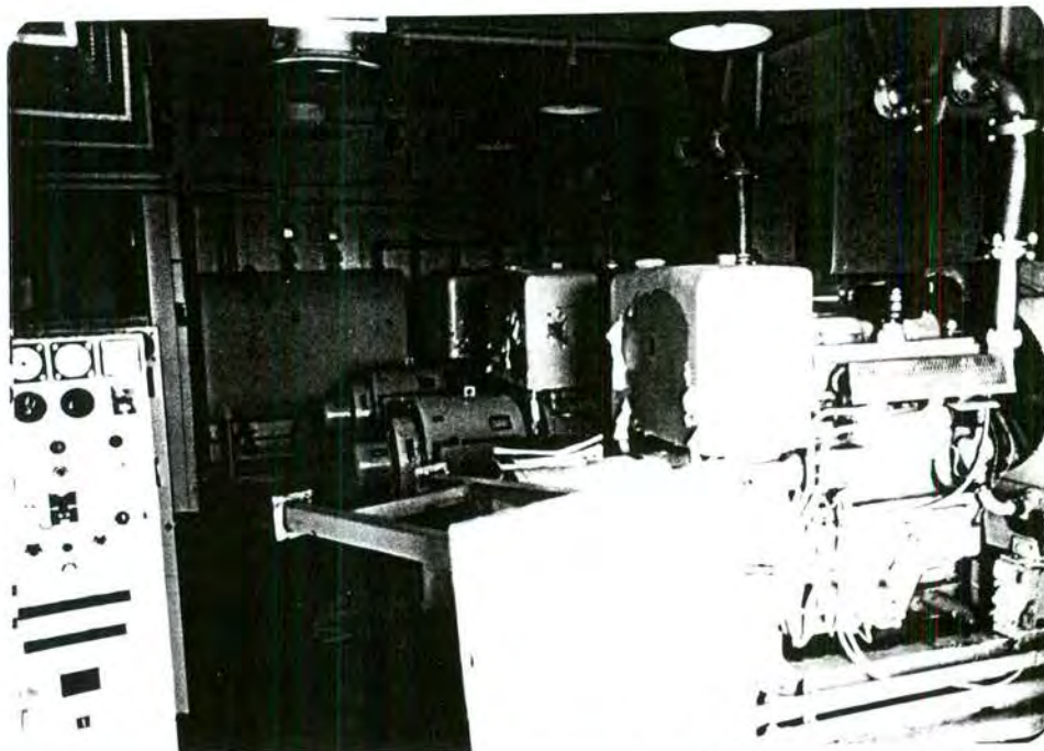
Photo 16: Three Dorman diesel generators in Doppler Detection Building at Site 306.
