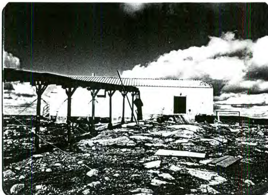
Photo 21: Highly scavenged Doppler Detection Building at Site 303.
